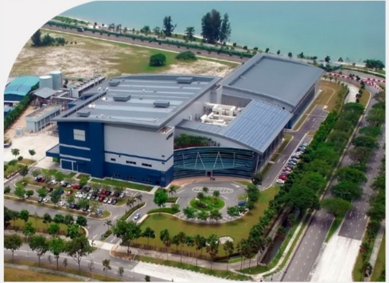
Lonza contract manufacturing facility in Singapore
