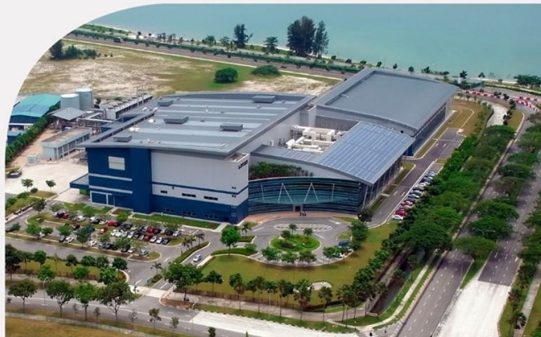
Lonza contract manufacturing facility in Singapore
