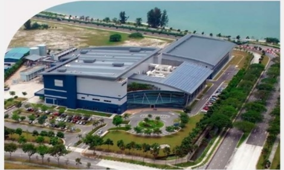
Lonza contract manufacturing facility in Singapore
