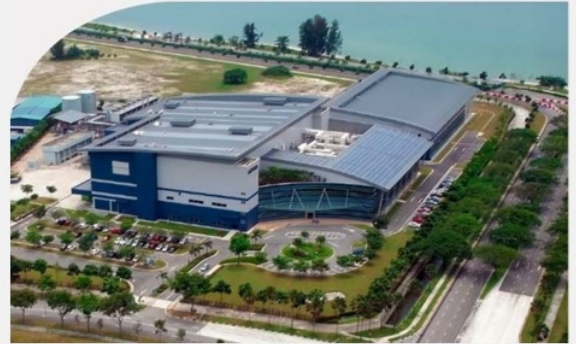
Lonza contract manufacturing facility in Singapore
