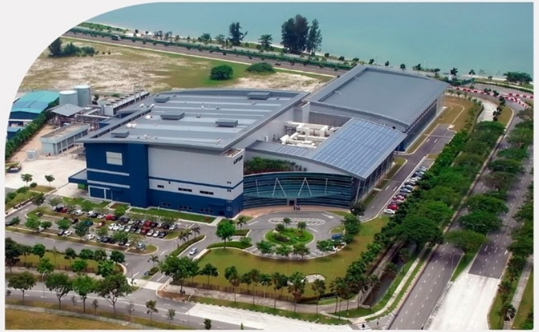
Lonza contract manufacturing facility in Singapore
