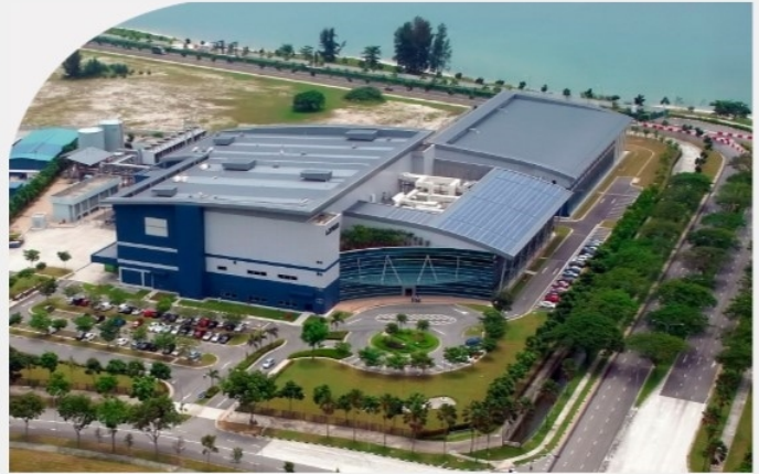
Lonza contract manufacturing facility in Singapore
