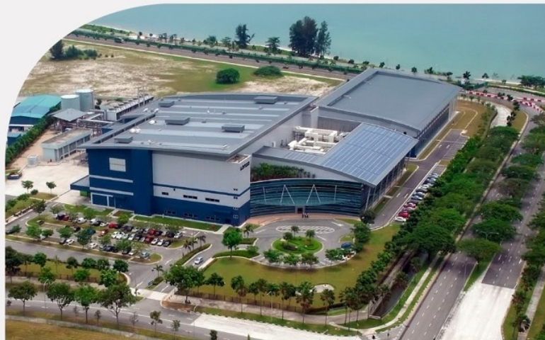
Lonza contract manufacturing facility in Singapore
